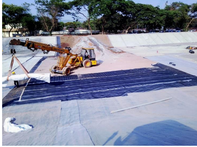
Laying of Geotextile layers
